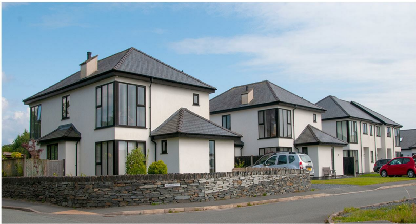
Cae Eithin, Morfa Bychan A development of 10 homes completed in August 2018
